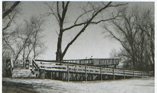
Eagle Lake, in Hancock County, has had a spectacular boardwalk/platform installed on the west side.
